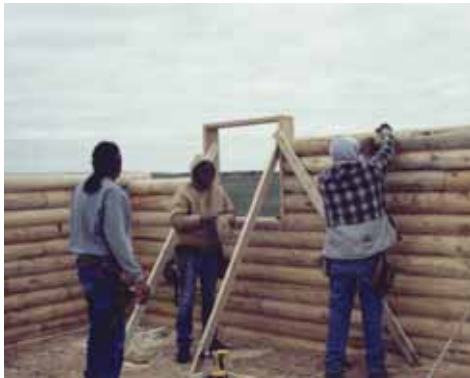
Members work together to build the house.
