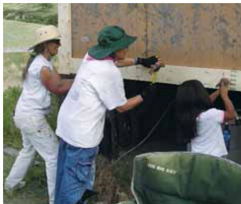
Candy Boyd, Ellen Daranowski, and Chante work on the house.
