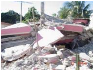
A for story apartment building in Port Au Prince, HAITI, destroyed by the January 12, 2010 earthquake.
